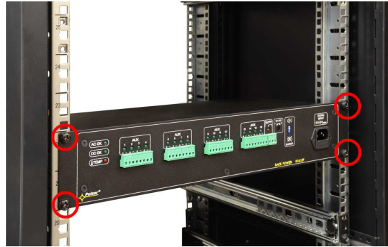
- Secure the enclosure with 4xM6 screws
